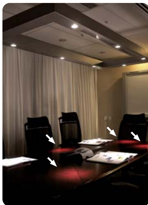
Meeting room illuminated by the LED GU10s that delivers spot illumination in dimmer environments.
